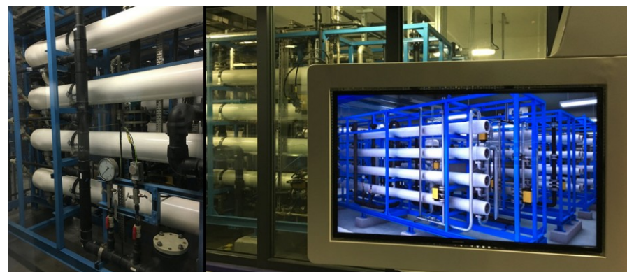
Figure 34 Advanced Reverse Osmosis Desalination Technology Source: Planning Department
